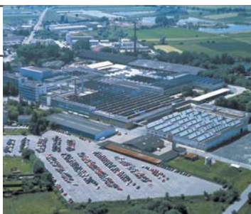
Stiebel Eltron's plant in Holzminden, Germany.
